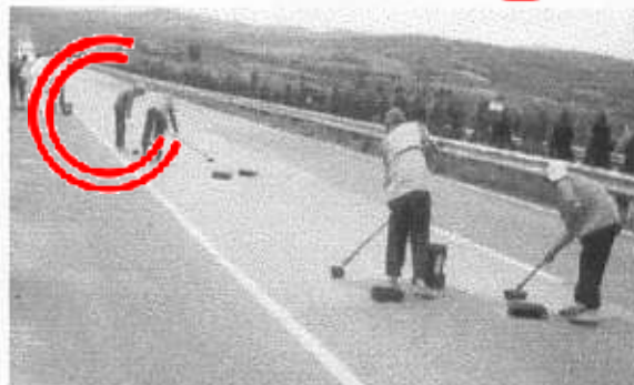
PHOTO 13 TYPICAL CHINESE REJUVASEAL DEMONSTRATION SECTION
