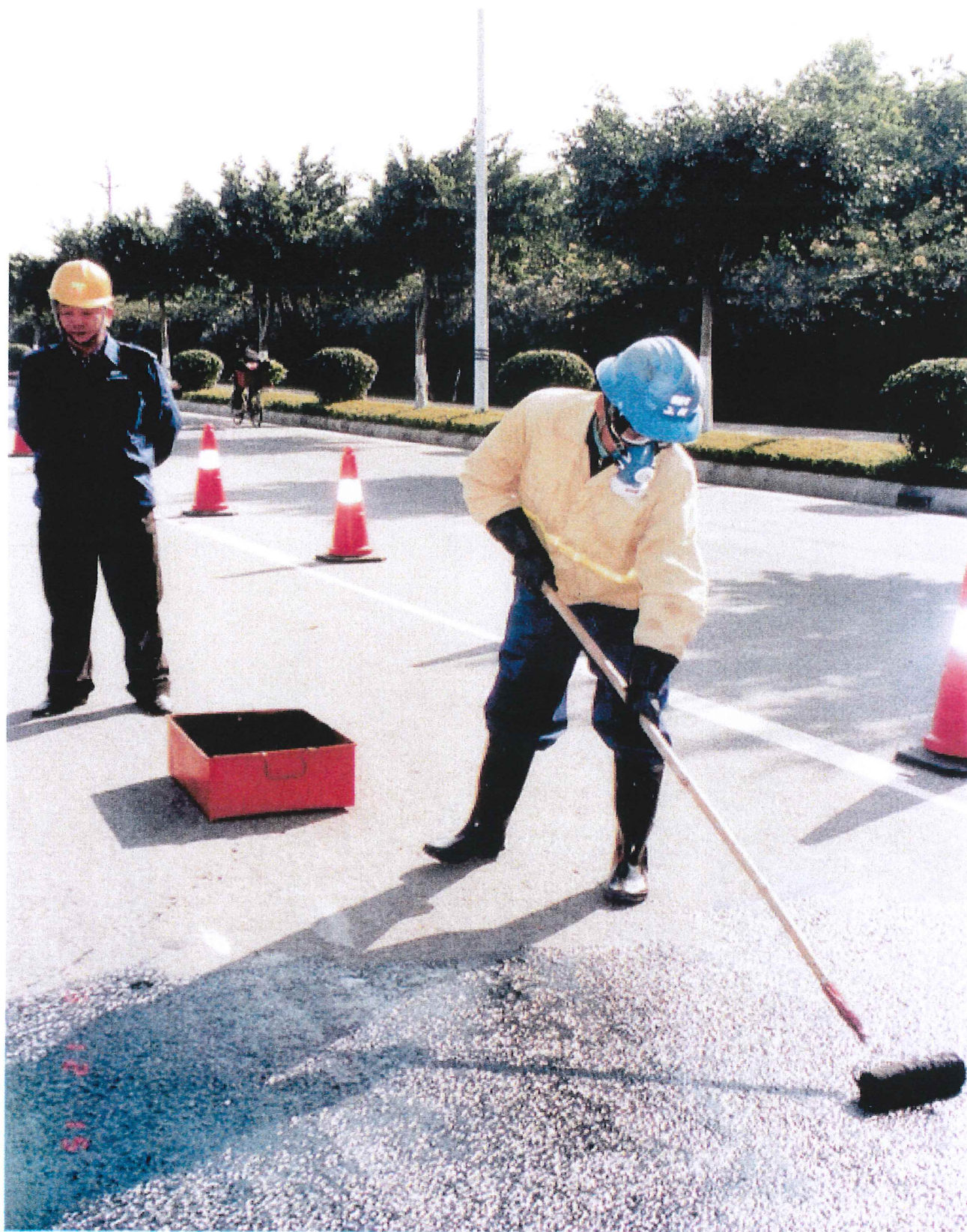
Figure 4.1 Typical Application Procedure for RJSeal.
