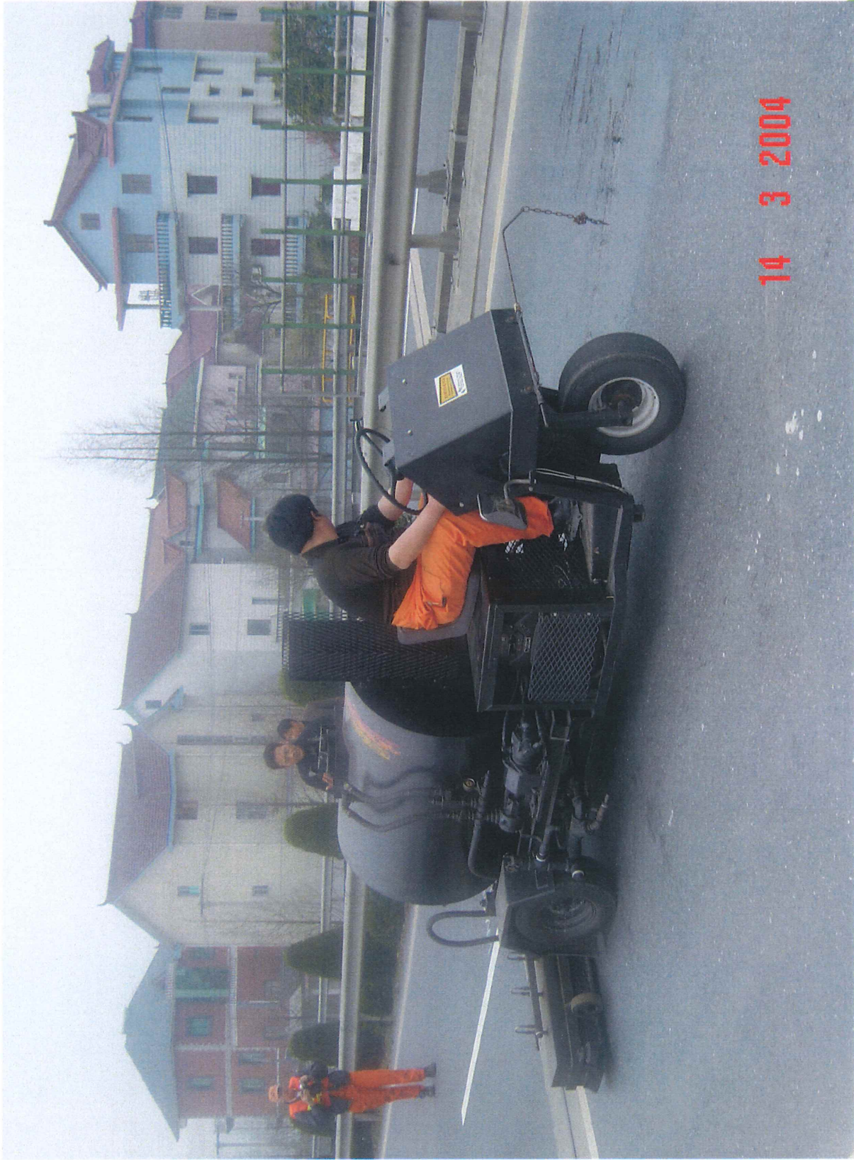
Figure 4.2 Typical Application Procedure for RJSeal
