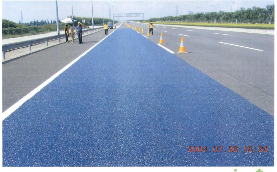
Figure 4.2 Finished RJSeal Surface.
