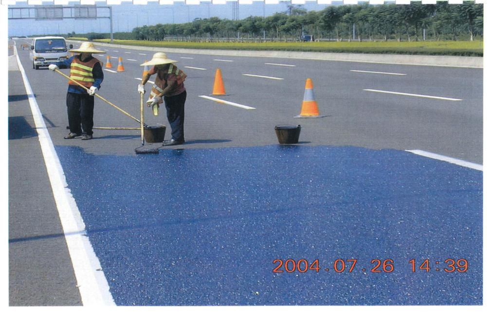
Figure 4.1 Typical Application Procedure for RJSeal.
