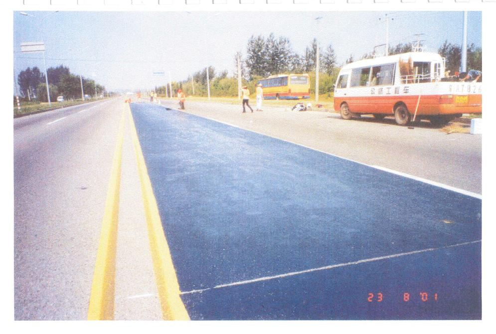
Figure 4.3: Finished Surface - RejuvaSeal TM
