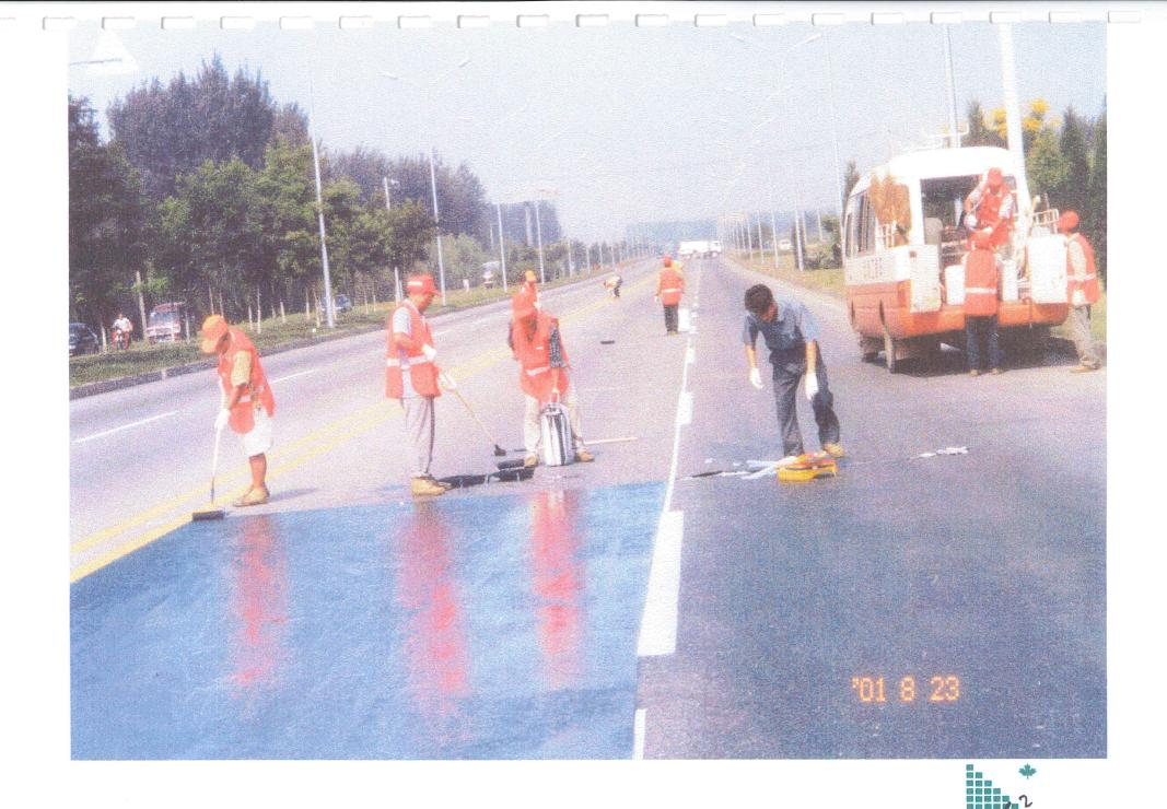
Figure 4.2: Typical Application Procedure for RejuvaSeal TM
