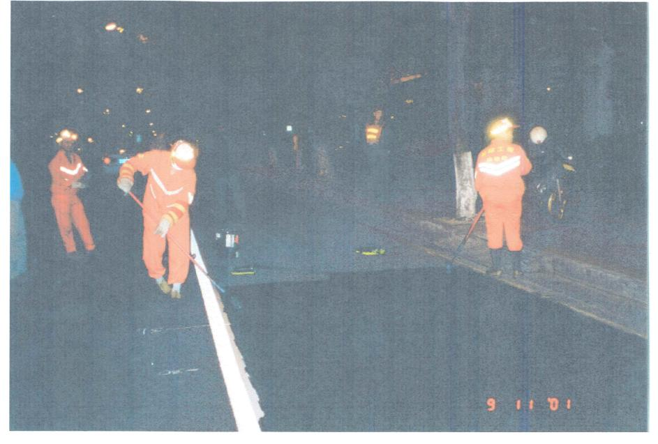
Figure 4.2: Typical Application Procedure for RejuvaSeal TM
