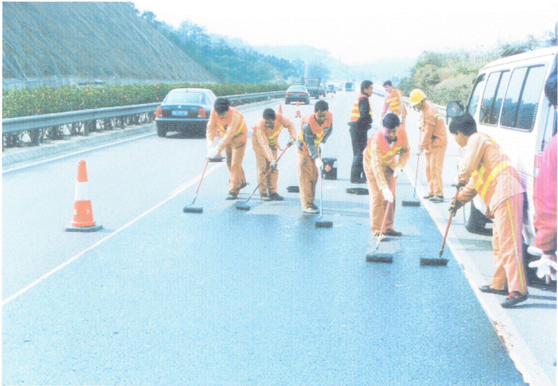
Figure 4.2: Typical Application Procedure for RejuvaSeal TM
