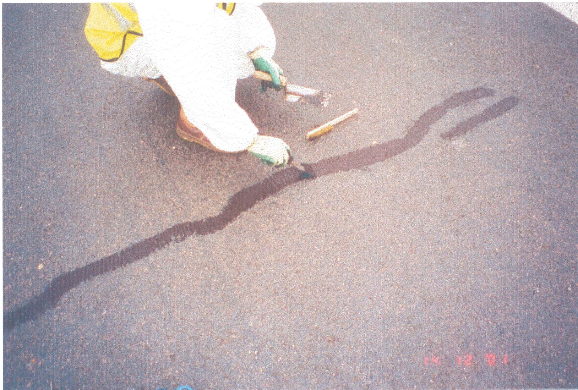
Figure 4.4: Cracks filled with crack sealant
