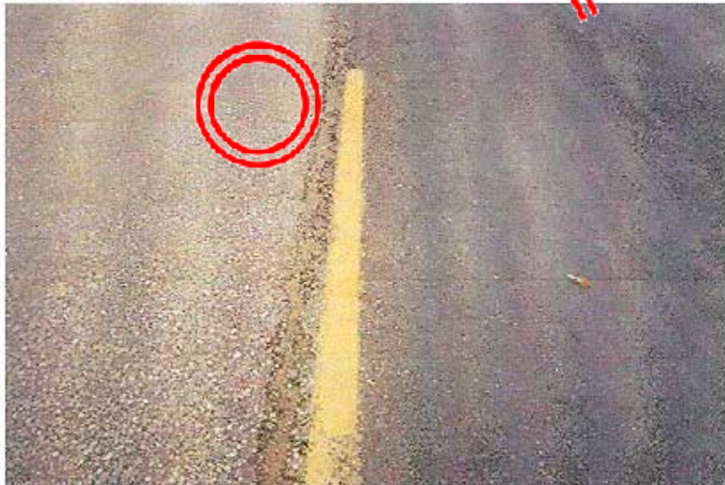
PHOTOGRAPH 8 Entwistle Sand RejuvaSeal Demonstration Project Performance October 2, 2000 [JJE]
