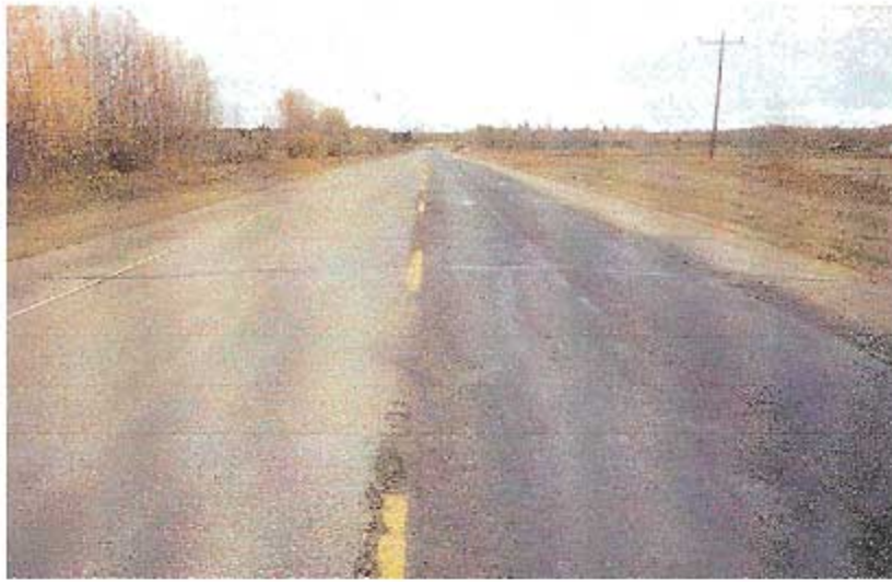
PHOTOGRAPH 7 Entwistle Sand RejuvaSeal Demonstration Project Performance October 2, 2000 [JJE]
